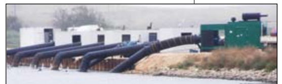
Temporary Weir at Narrung Narrows
